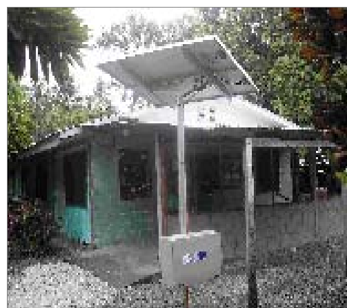
Household solar PV system Installed at Jeh, Ailinglaplap Atoll
