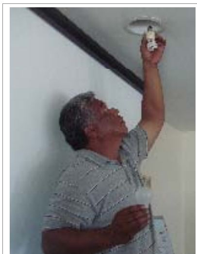
Replacing inefficient light bulb with a compact fluorescent light
